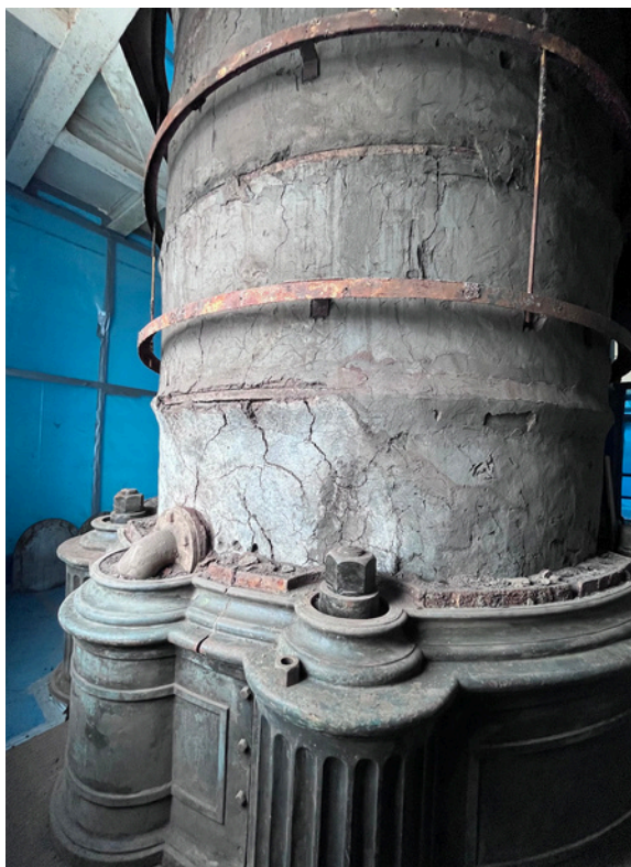
Lagging sheets removed, original lagging still in place.
