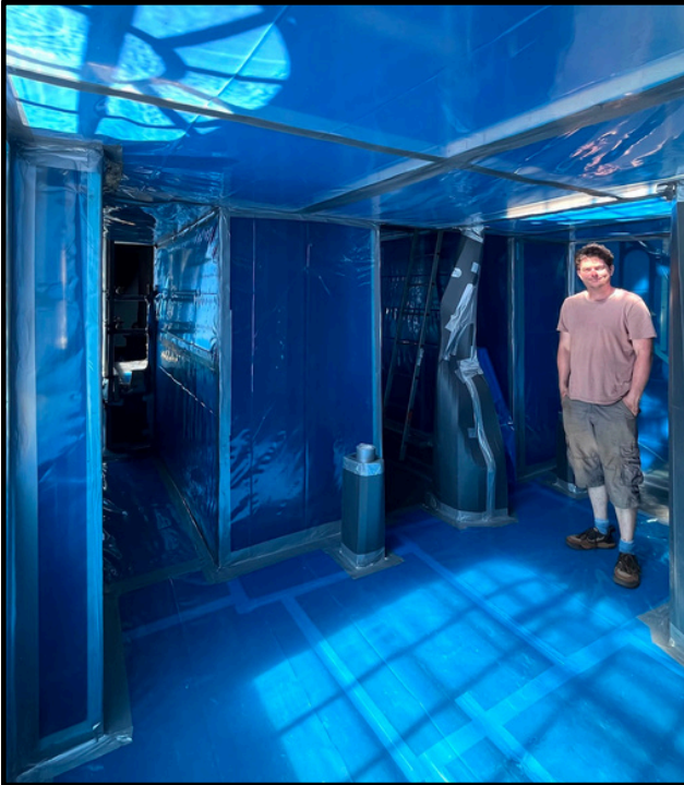
Glen standing in the Great Engine House that is covered in scaffolding and polythene sheeting prior to works.
