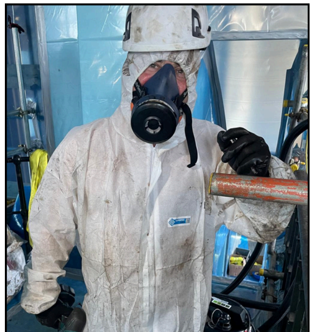
Richard halfway through a very warm day of work removing asbestos.
