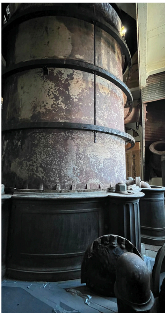
Lagging sheets removed, lagging removed.
