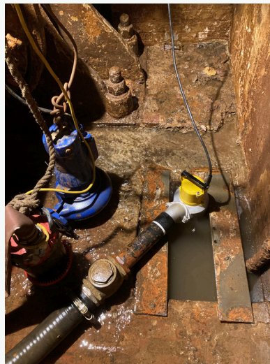
New WEDA submersible Pump for Bull engine supplied by Trebles
