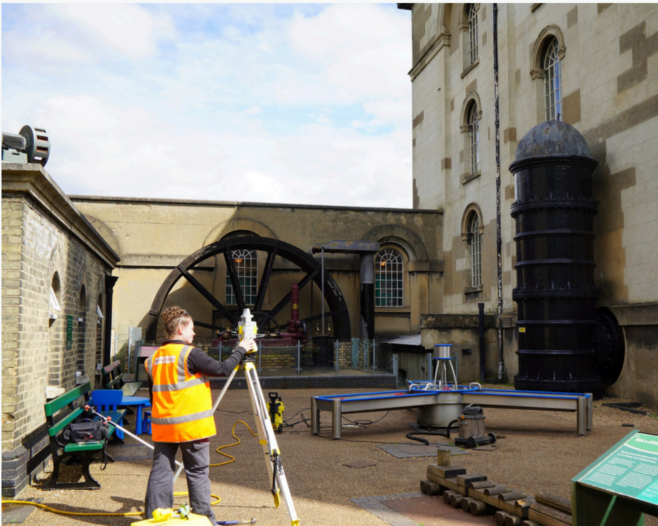
Topographical survey in progress.
