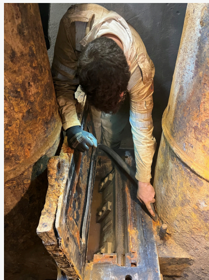
Volunteer Richard dismantling non return valve
