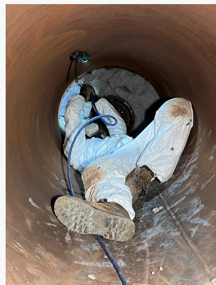
Dal from Heatbox Engineering inside the boiler.
