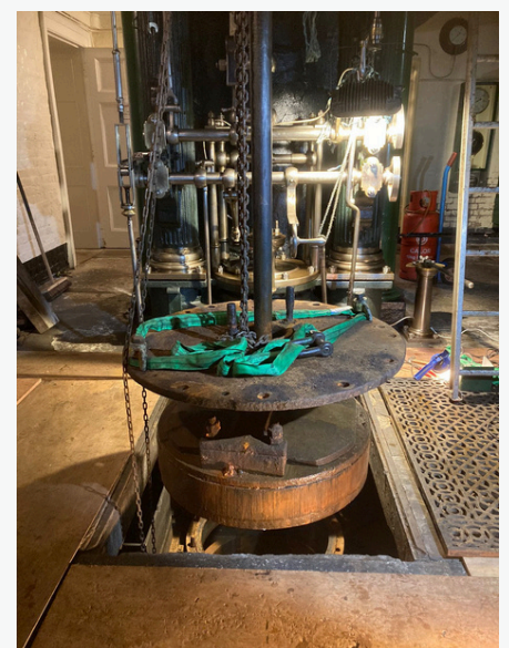
Figures 1 & 2 & 3: air pump dismantling, unbolting air pump top cover, removing air pump piston
