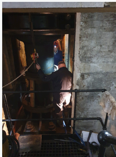
Clive Penfold and Tim Wellburn on pump gland repacking the Bull Engine
