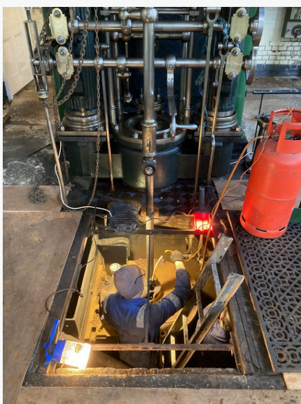
Figures 1 & 2 & 3: air pump dismantling, unbolting air pump top cover, removing air pump piston
