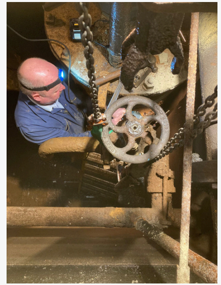
Figure 6: Clive Penfold preparing to cut off bolts to condenser cooling water valve to B&W
