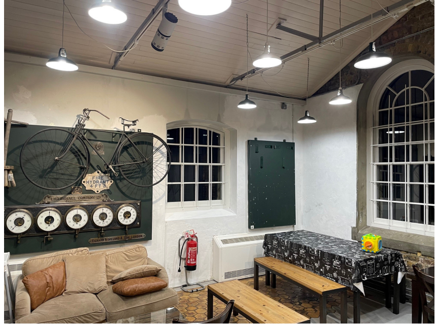
Repaired plasterwork in the cafe
