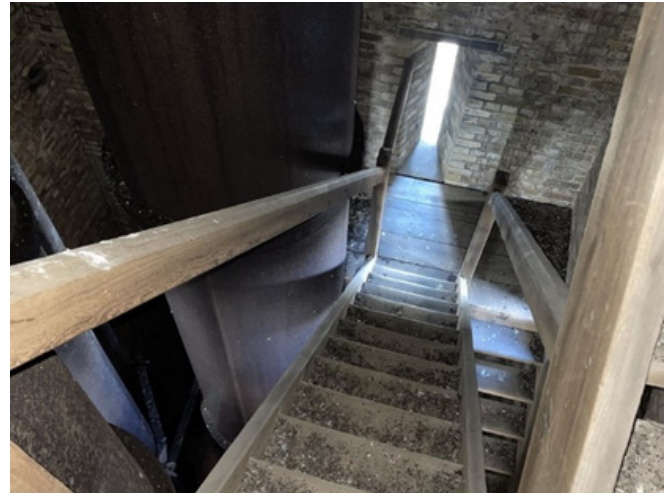
View down the stairs inside the tower
