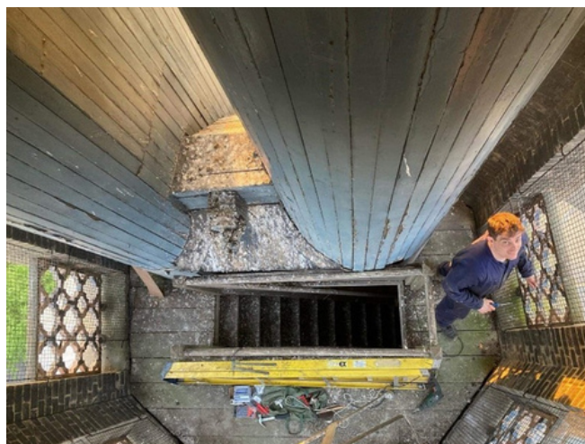
Repairing mesh screens inside the tower
