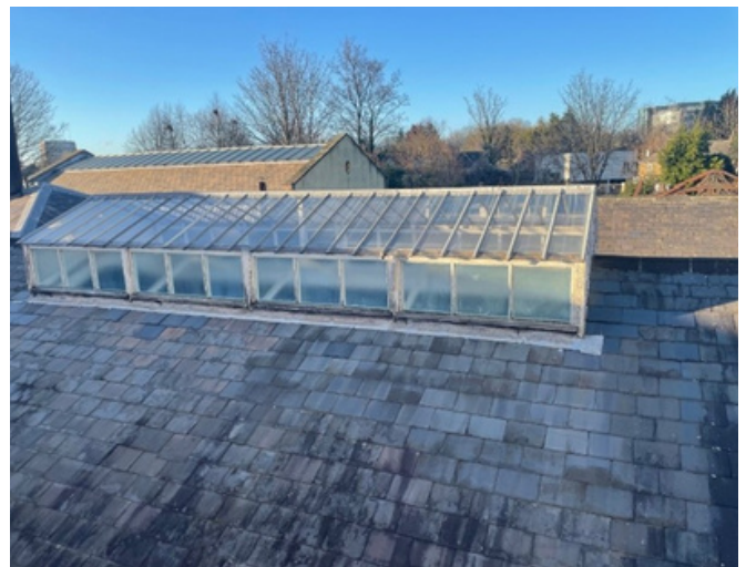
View of the Steam Hall skylight
