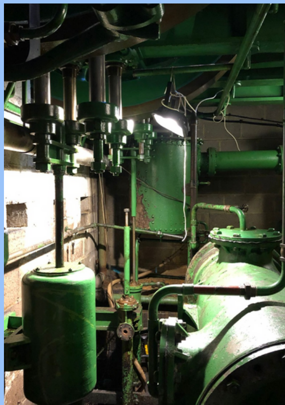
The basement under the Triple
